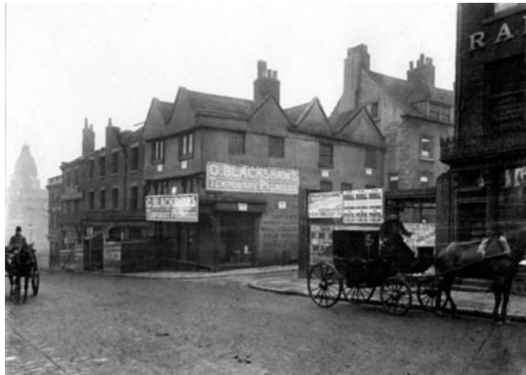
Timber framed house on the corner of Change Alley and High Street (demolished in 1895 to allow for road widening).
