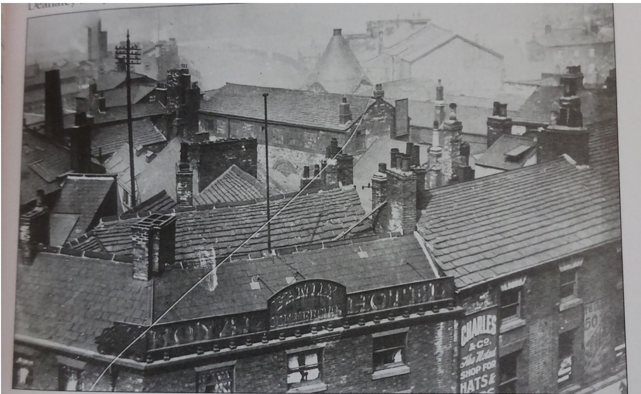
From the roof of Davy's restaurant on Haymarket, looking towards the Royal Victoria Hotel before the area was redeveloped in 1914-20. The view is of historical interest as it shows the site of the medieval castle, subsequently covered by a jumble of property including the cone of an early steel cementation furnace.
