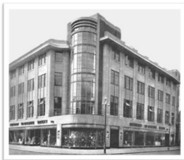
Figure 3: Co-operative society's Emporium, "Beacon house", Southport (Co-operative News, 1935)
