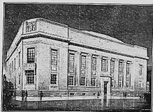
The Direct Labour Department made this beautiful addition to Sheffield's architecture. It serves the student, the ordinary reader, and the child. The special Art Gallery presented by Alderman Graves is on the upper floor.
